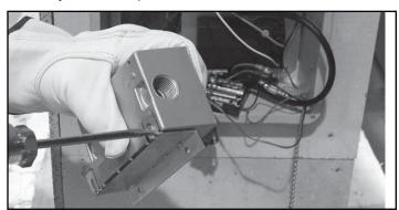
Figure 6.7 Fasten Bracket to Junction Box
